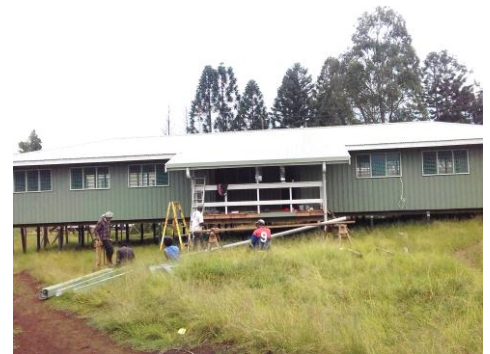
Above: Double classrooms near girl's dorm. Below: Dorm up-lifting, Admin extension.
